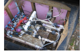
Plug and Play: valves, meter, filters and heater
